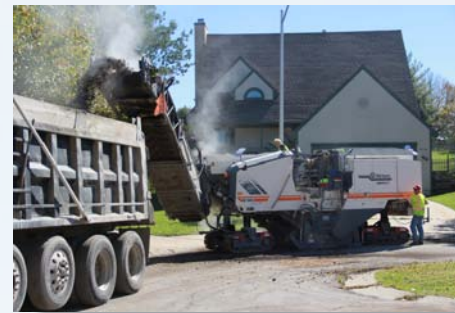
Part of the KCMO overlay project was milling and repaving neighborhood streets.
