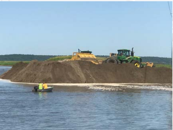
The scour hole was over 50 foot deep when crews started. Over 311,000 cubic yards of dirt had to be moved to fill the hole and rebuild the levee.
